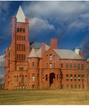
Pillar of Fire
